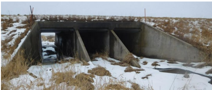
Concrete Box Culvert
