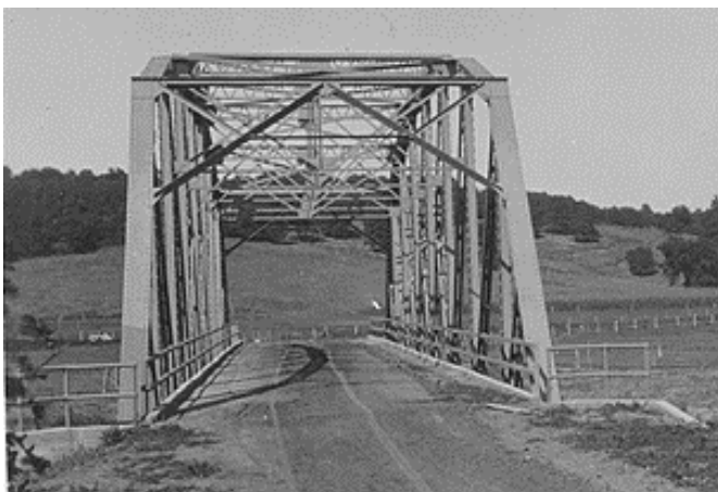
Steel Thru Truss
