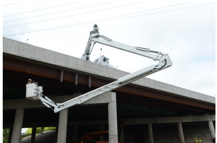
Under Bridge Inspection Vehicle
