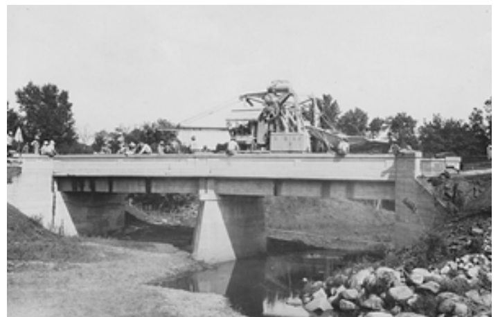
Early 1900's Bridge Construction
